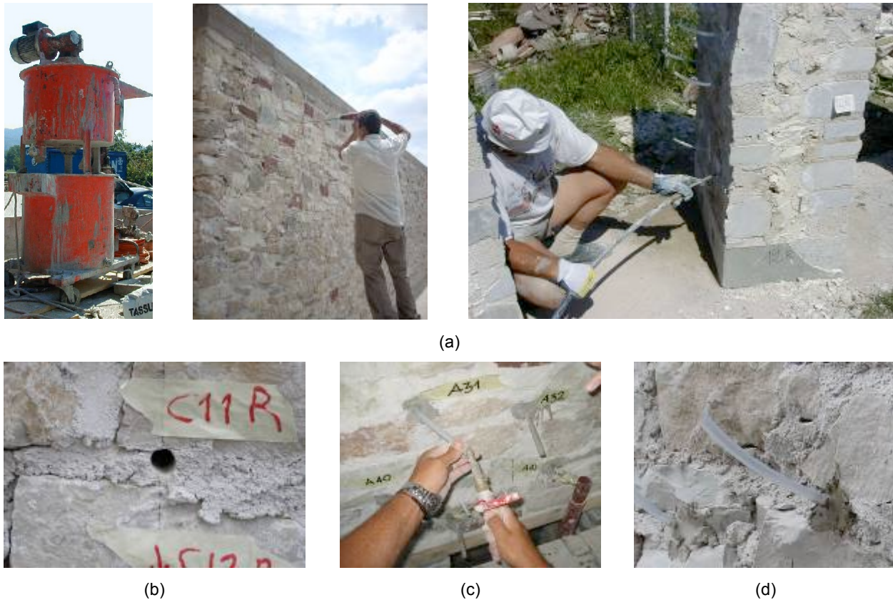
Figure 3.4 Grout injection procedure. (a) General overview of the process. (b) Drilling holes in mortar joints. (c) Fixing plastic pipes. (d) Injecting grout (Source: UNIPD).
