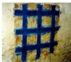
Figure 3.42 Layout of a FRP reinforcing.
