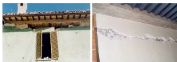
Figure 4.6 Difficult connection between the tie beams and the walls.
