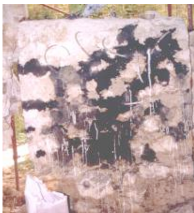
Figure 3.18 Filling of the cracks, (Binda et al., 2005).
