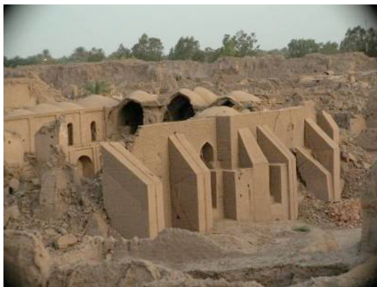
Figure 3.67 Collapse of domes adjacent to newly built buttresses, (Source: Randolph Langenbach).
