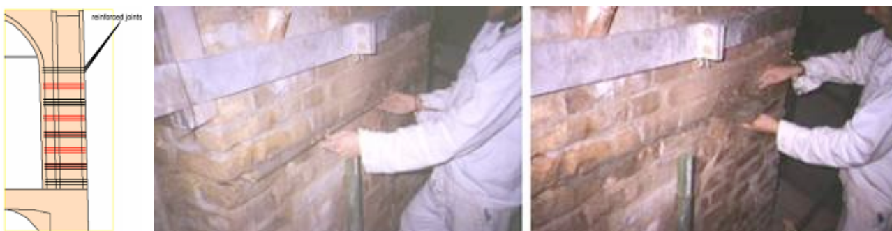
Figure 3.46 Bed joint reinforcing of a compressed pillar, (Source: UNIPD).
