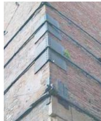
Figure 4.17 External confinement by metal tie, (Source: UNIPD).
