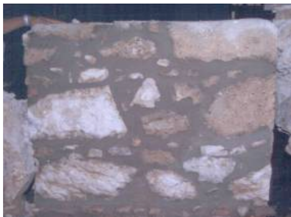
Figure 3.21 Repointing, (Binda et al., 2005).
