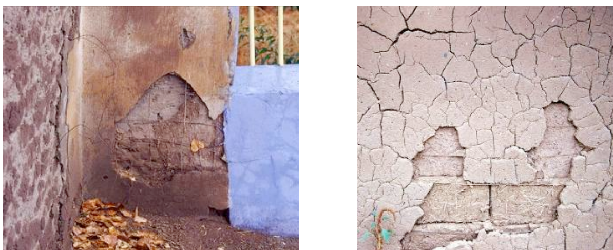
Figure 3.14 Cracking and spalling of earthen mortar over steel mesh reinforcement, Chile (Source: BAM).
