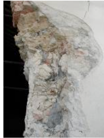
Figure 3.3 Only some spots were injected in the case of this wall with a very low percentage of voids, (Binda et al., 2003a).
