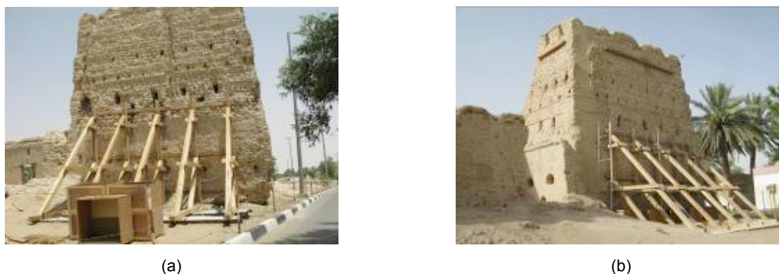
Figure 3.52 Application of the “scuci-cuci” technique to the gate at Al Damarki as crack repair, (source: ZRS).
