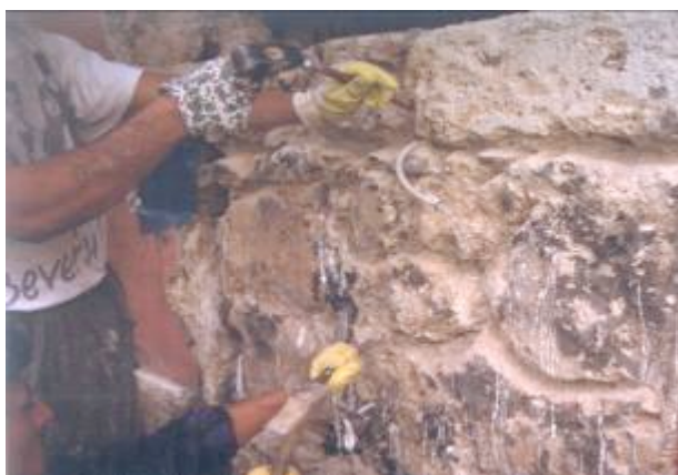
Figure 3.19 Cleaning of the joint up to 70.0mm, (Binda et al., 2005).
