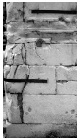
Figure 3.57 Crack stitching by metal bars, (Source: POLIMI).
