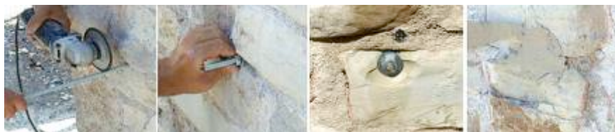
Figure 3.41 Positioning of anti-expulsion tie-rods.
