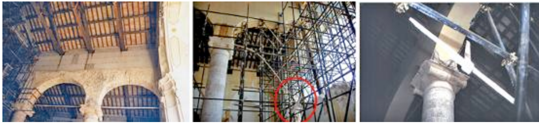
Figure 4.16 The tie was not able to restraint the wall overturning; the stiff and heavy R.C. tie beam pushed over the church façade, (Source: POLIMI).
