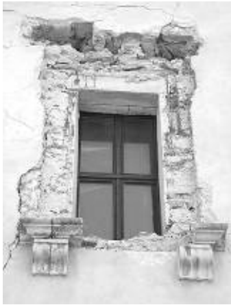
Figure 3.2 Poor results of applied injection, (Binda et al., 2003a).
