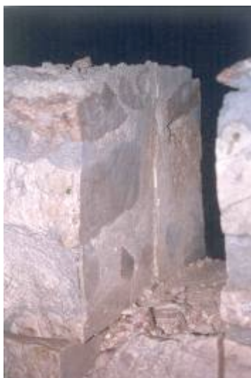
Figure 3.27 A cut section of the repointed wall, (Binda et al., 2005) and (Corradi 2008).
