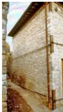
Figure 4.17 External confinement by metal tie, (Source: UNIPD).
