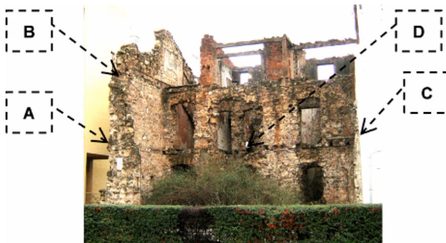
Figure 4.18 Residential Building Bulevar 25 in Mostar, Bosnia and Herzegovina. Position of visible metal ties marked A to D. Front facade wall demolished above the ground level. Photo Interprojekt, December 2009.
