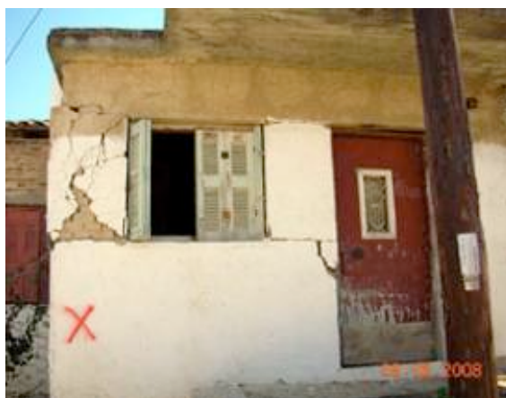
Figure 4.8 A R.C. tie beam is constructed over the opening. Disintegration of the pier and horizontal sliding is observed, (Source: NTUA).
