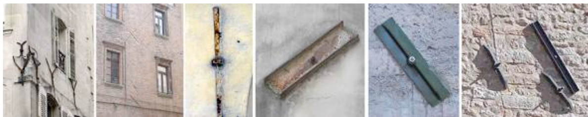
Figure 4.14 Example of tie anchors.
