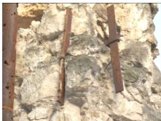
Figure 4.19 Residential Building Bulevar 25 in Mostar, Bosnia and Herzegovina. Detail A. Detail of the anchors on the facade. Photo Interprojekt, February 2009.
