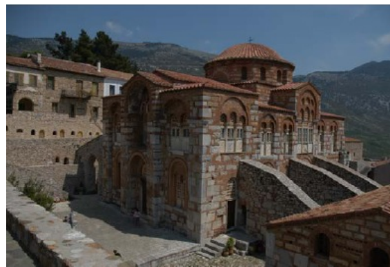
Figure 3.64 Katholikon of Ossiou Lucas Monastery-Added buttresses (south façade), (Source: NTUA).
